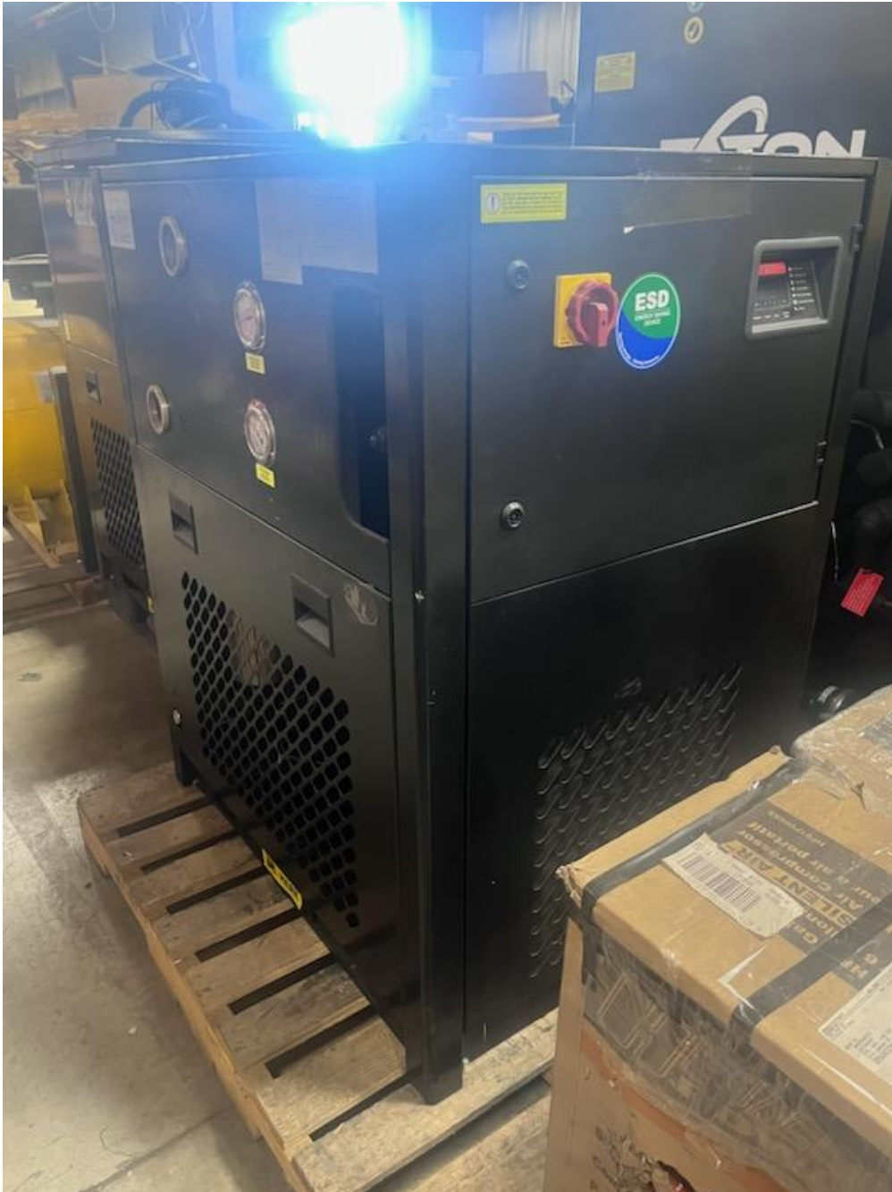
S&D POLAR 288CFM 3 PHASE 460 VOLT DRYER
